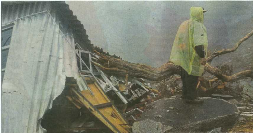
Heavy losses: The Laban Rata hostel on Mt Kinabalu was badly damaged during the June 5 earthquake.
